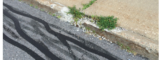
PDE pavement that will be replaced
